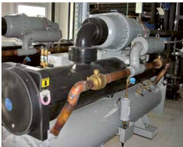
In Hungary, our Zalaszentgrót plant recovers heat energy from natural springs, reducing the plant's natural gas usage by 60%.
